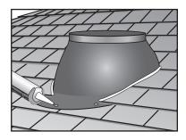
**STEP 12** Peel the protective backing off the black horse hair gasket (C) and apply gasket on the inner lip of the flashing collar (E).
