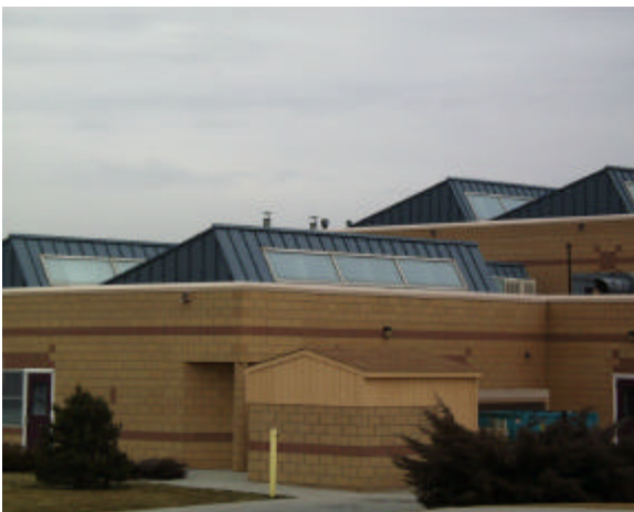
Figure 7: New Fort Collins School with Monitor Skylights
