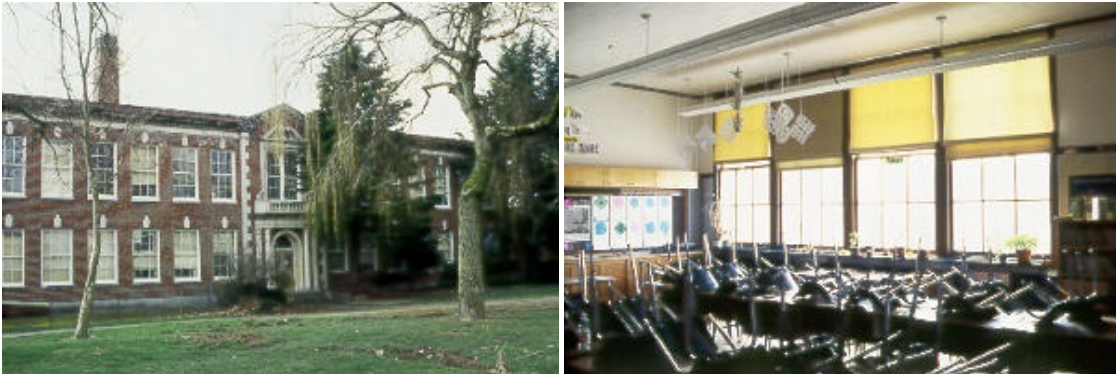
Figure 5: Older Seattle School With Windows Code 4, Exterior (left), Interior (right)
